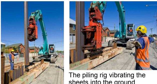
The piling rig vibrating the sheets into the ground
